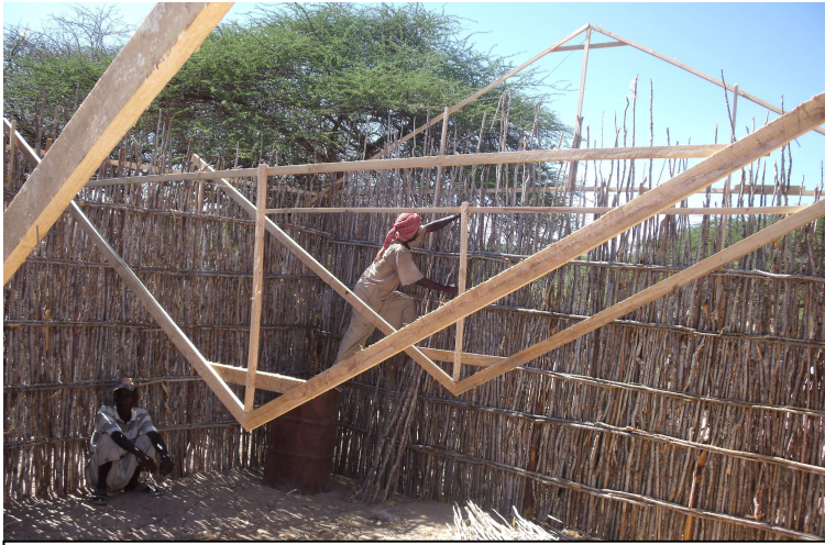
Qasab2 Camp learning center construction is carrying on.
